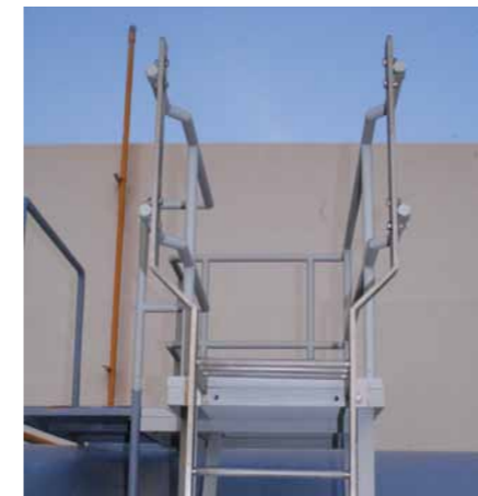
Painted Steel Platform
