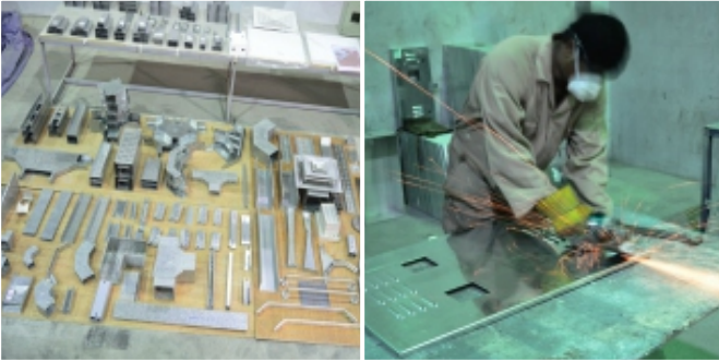
All type of steel fabrication work
