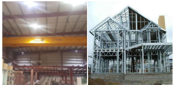
QT works on steel frame factory and house, factory required Crane.
